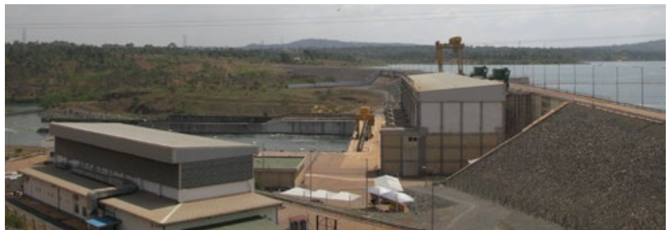
The Bujagali hydropower plant in Uganda (CAO).
