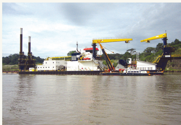
Panama Canal Expansion Project, Panama.
