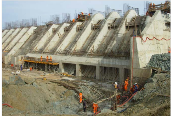
View of the Bujagali power plant during construction
