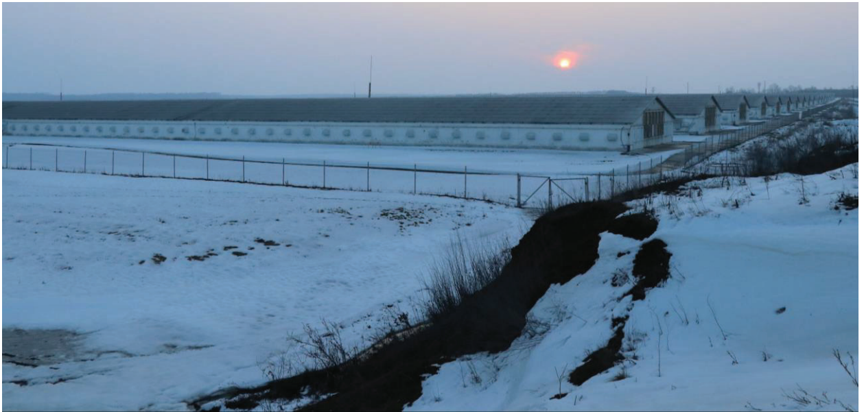
Existing poultry houses within the VPF.
